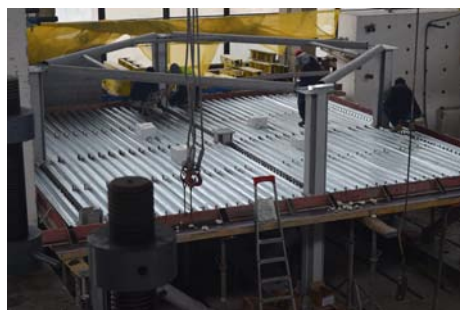
Fig. 6. Composite slab system during construction
